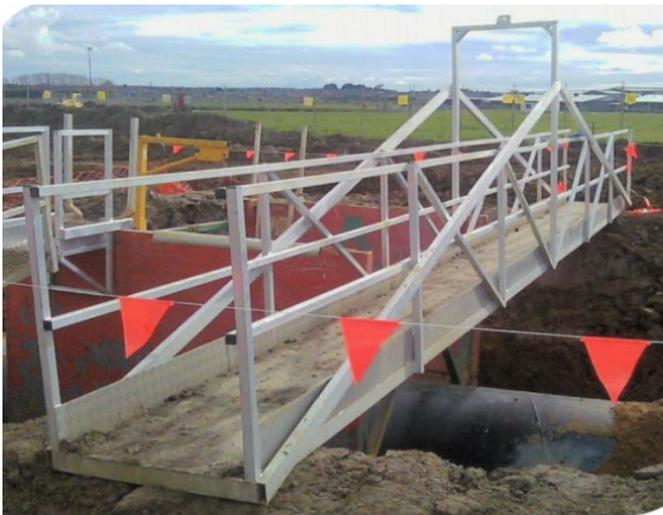
12. Fall protection - Where personnel and/or equipment must cross an excavation, a walkway or bridge with appropriate guardrails should be engineered to withstand the maximum expected load. All excavations in a remote or unattended location should have adequate barriers or physical protection to prevent people from falling into the excavation. Upon completion, back fill all trenches, wells, pits, or shafts as soon as practical.
