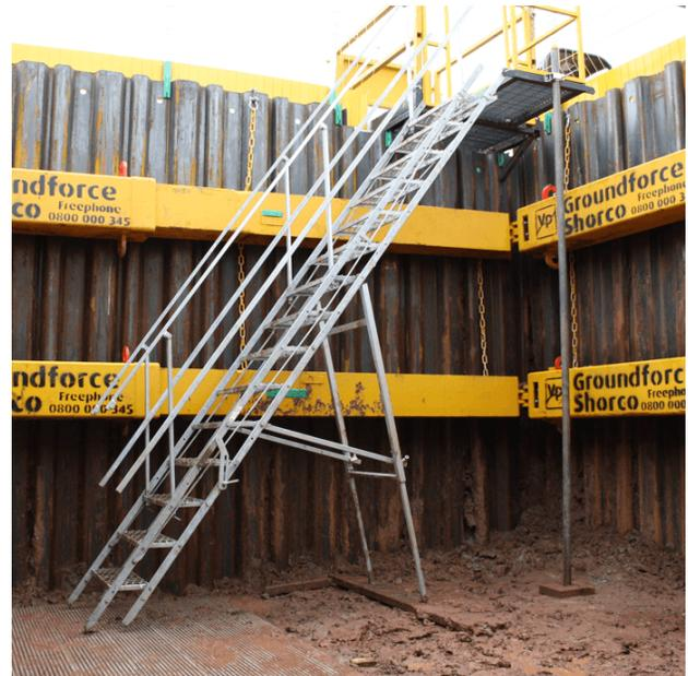
3. **Access and egress** (entrance and exit) - Any trench or excavation four feet or deeper should have a means of exit. Ladders and/or ramps are best located no more than twenty-five feet in any direction. Ladders should extend three feet above the surface of the excavation and be tied off if necessary.
