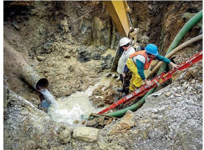
8. Hazards associated with water accumulation - Workers shouldn't work in excavations where water is accumulating unless adequate precautions are taken to protect from these hazards. This protection involves specific shoring, pumping, and well points for water removal, and careful monitoring by a competent person.
